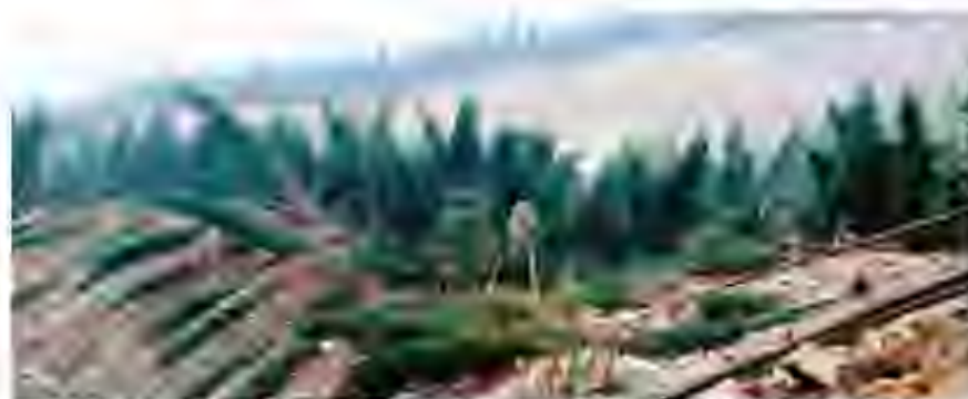
Figure 3.1. Deep seated landslide resulting from the 2008 Sichuan earthquake. Trees had no mitigating effect Courtesy: Patrick Duret.
