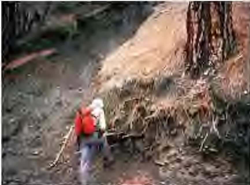
Figure 2.4. Ponderosa pine tree buttressing a slope above a forest road. The unprotected portion of road cut to the left has fallen. Mendocino National Forest, California, 1978
