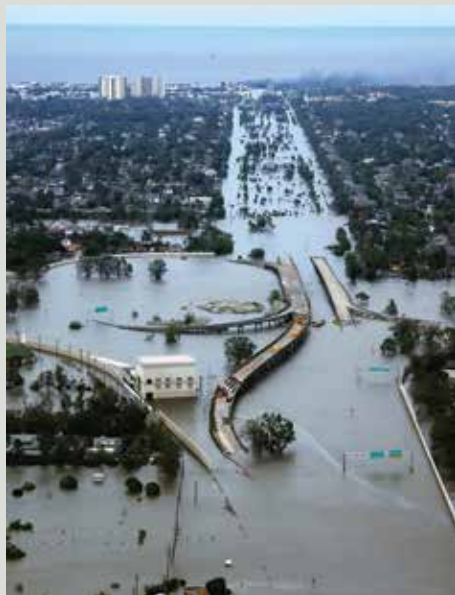
Left: Aftermath of 2005 Hurricane Katrina in New Orleans.
