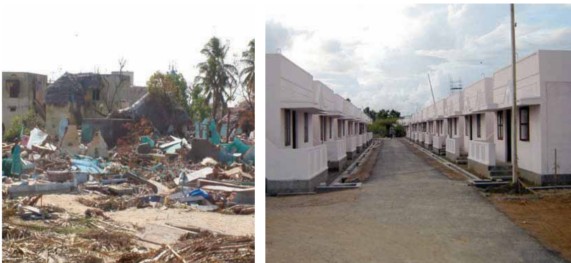
Damaged Houses, (December 2004) and Reconstruction of houses, Nagapattinam, Tamil Nadu (September 2005)
