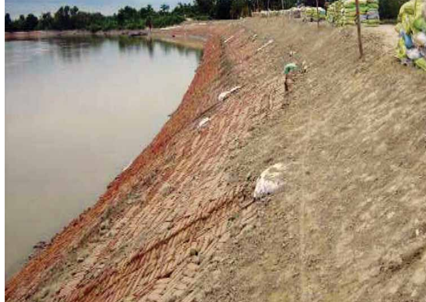
Raising & strengthening of Embankment on River, Burhi Gandak
