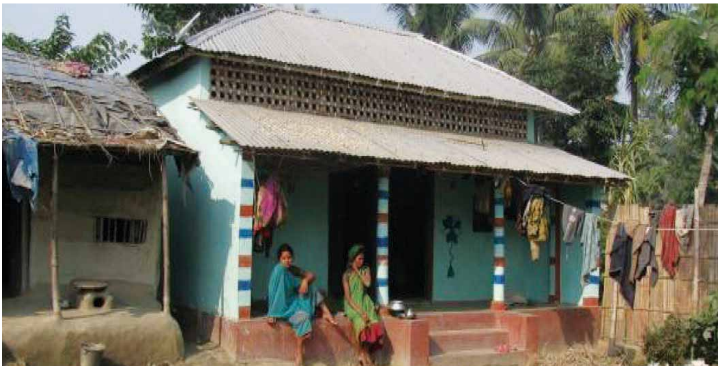
Owner driven construction under Kosi recovery programme
