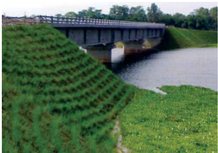
Doria Bridge, Assam, India
