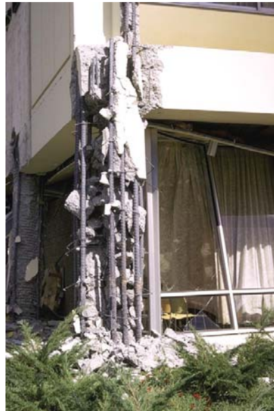
an earthquake damaged non-ductile reinforced concrete column (1971 San Fernando Earthquake)
