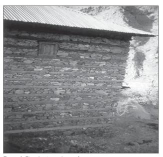
Figure 3. Zinc sheets used as roof
