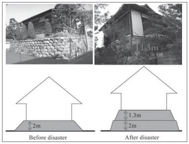
Figure 6. The Mizuya's plinth height was increased after the 1896 flood disaster (Photo by NIED-KU, 2007)
