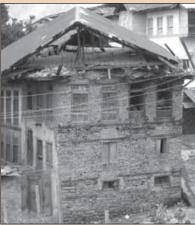
Figure 3. a) Portions where Dhajji-Dewari system (gable portion) and b) Taq system (entire structure except gable portion) survived the destruction of the 2005 earthquake.
