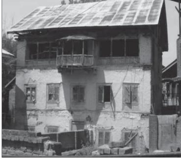
Figure 1. Houses with typical Taq type construction in Srinagar. Photo: Amir Ali Khan
