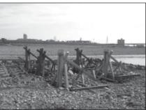
Figure 3. Hijiri-ushi made of concrete (Photo by NIED-KU, 2007)
