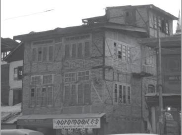
Figure 2. Houses with typical Dhajji-Dewari system of construction in Srinagar. Photo: Amir Ali Khan
