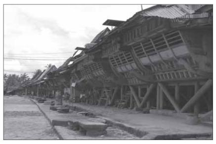
Figure 3. The traditional house in Nias, a time-tested and effective earthquake resistant structure.
