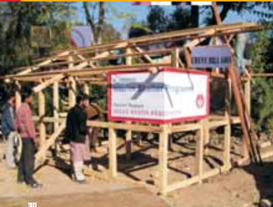
Safe Construction Practices : Interim Shelter in Poonch, Jammu & Kashmir
