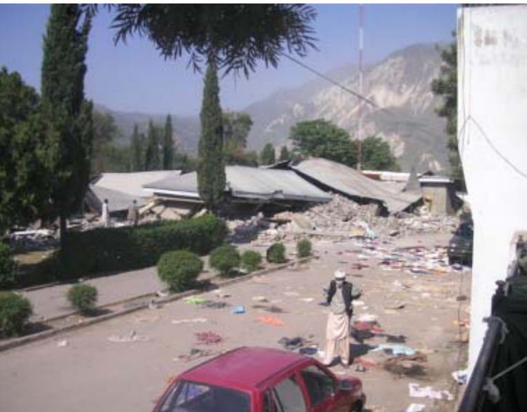
Collapsed public infrastructure (Photo credit: Roger Yates)
