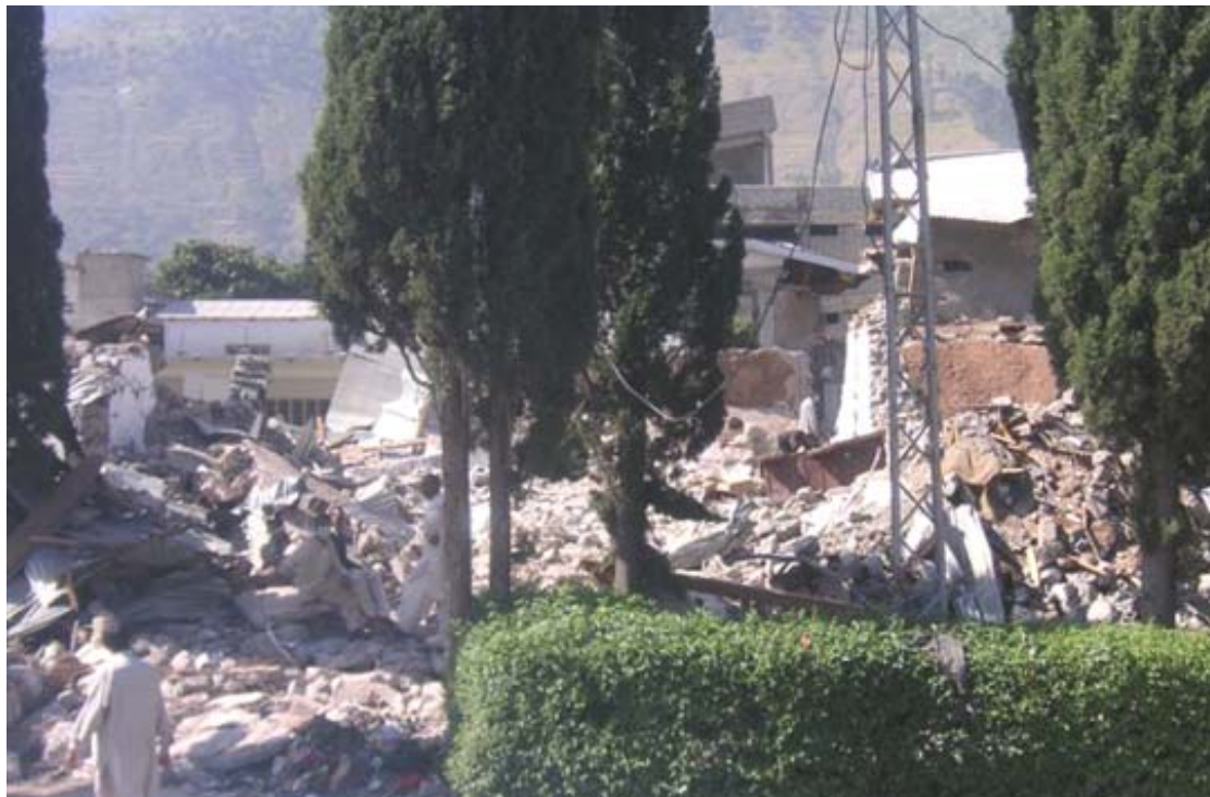
Collapsed public infrastructure (Photo credit: Roger Yates)
