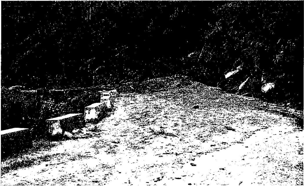
Fig. 5 Debris deposit on Trashigang –Mongar Highway due to flashflood (DoR)
