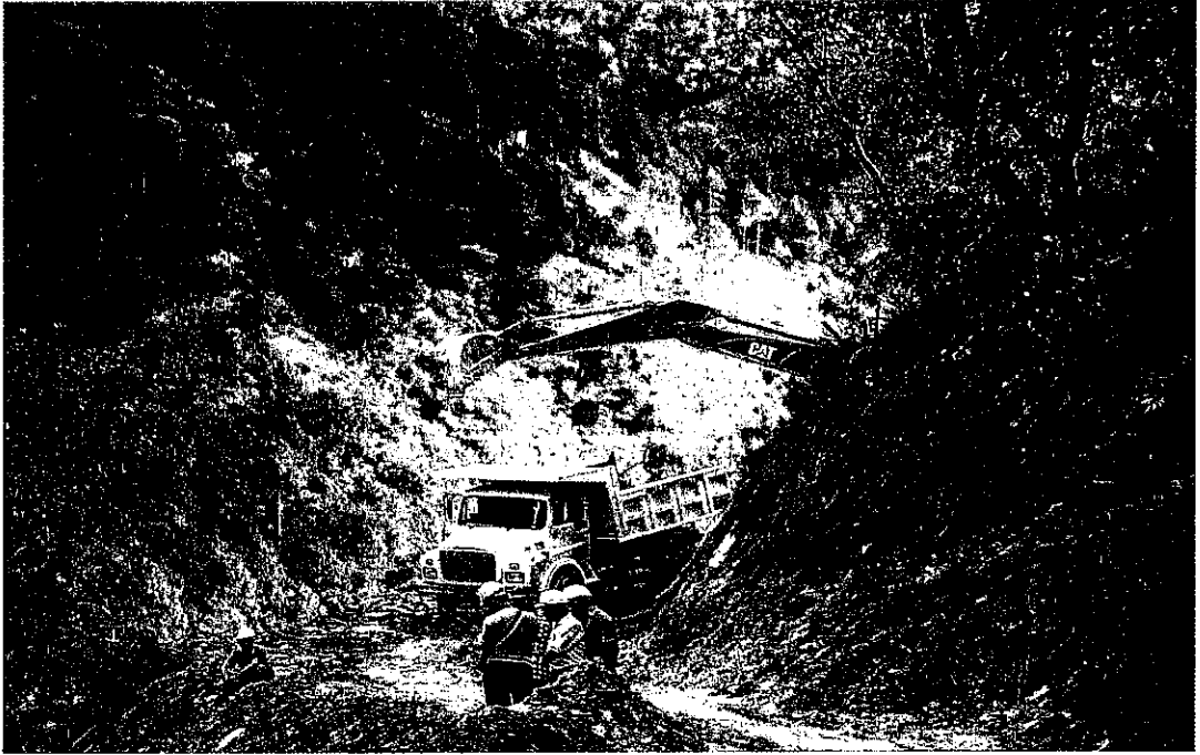
Fig. 7 EFRC method of road construction in Yadi-Sershong road (Pema Dorji)
