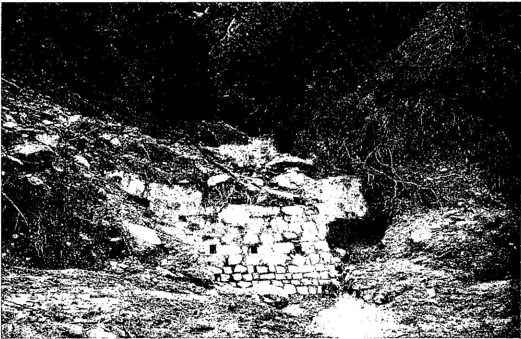
Fig. 6 Flashflood damaging permanent civil structures in the East (DoR)
