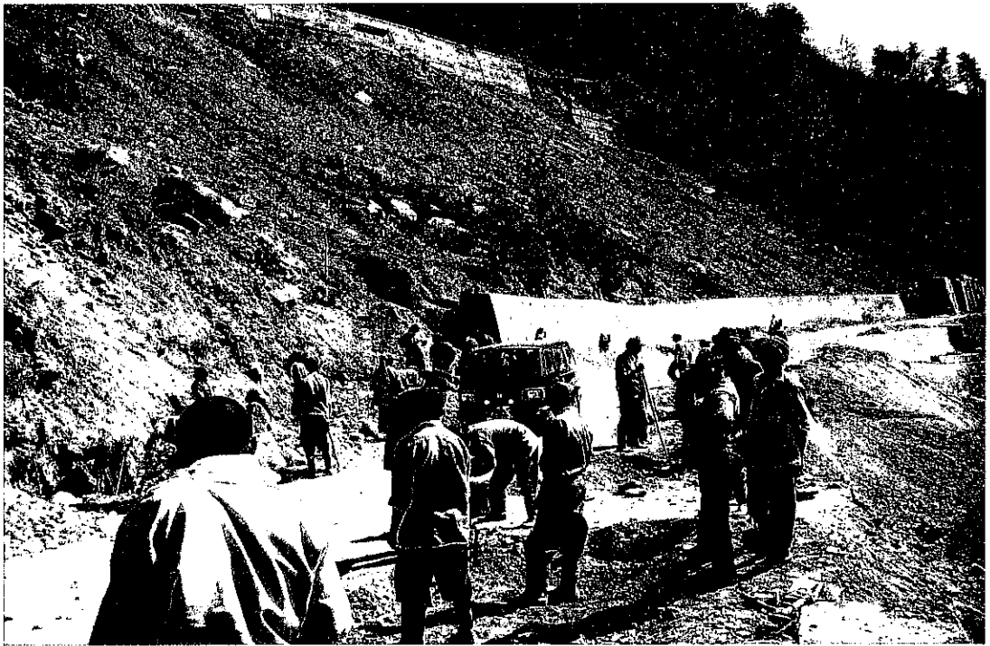
Fig. 6 Sorchen landslide in phuentsholing- Thimphu highway.
