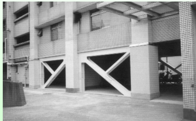
Example 1 of reinforcement of pilings
