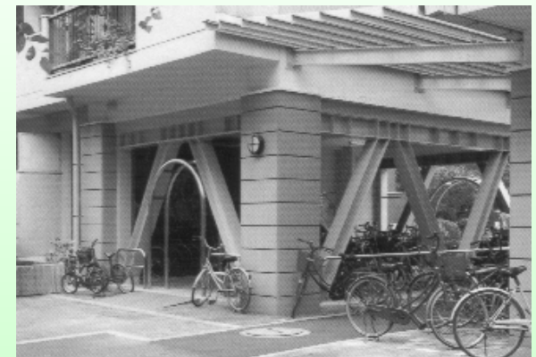
Example 2 of reinforcement of pilings
