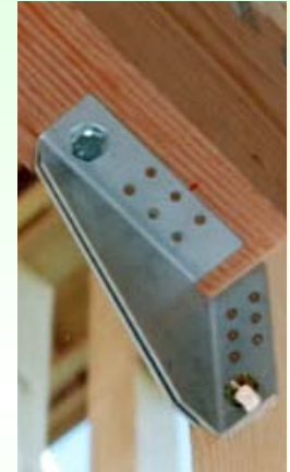
Damper hardware for seismic control
