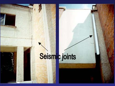
Improper or seismic joints
