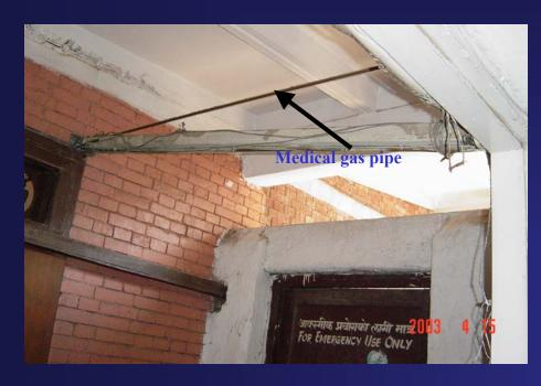
No extra precaution for passing the medical gas pipe from one building to another, no flexible coupling.
