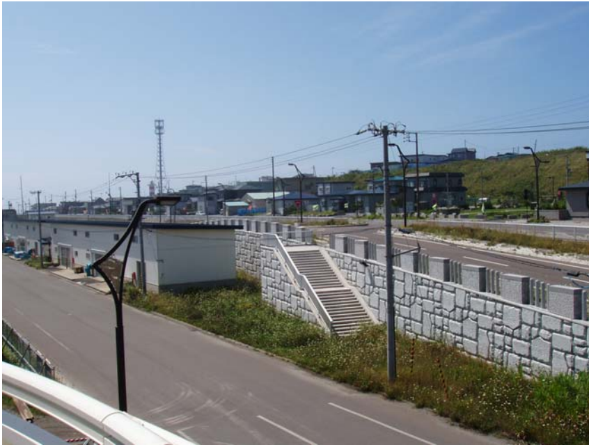
Fullfill mound and seawall Cooperative shed
