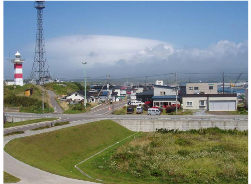
fill mound and high ground
