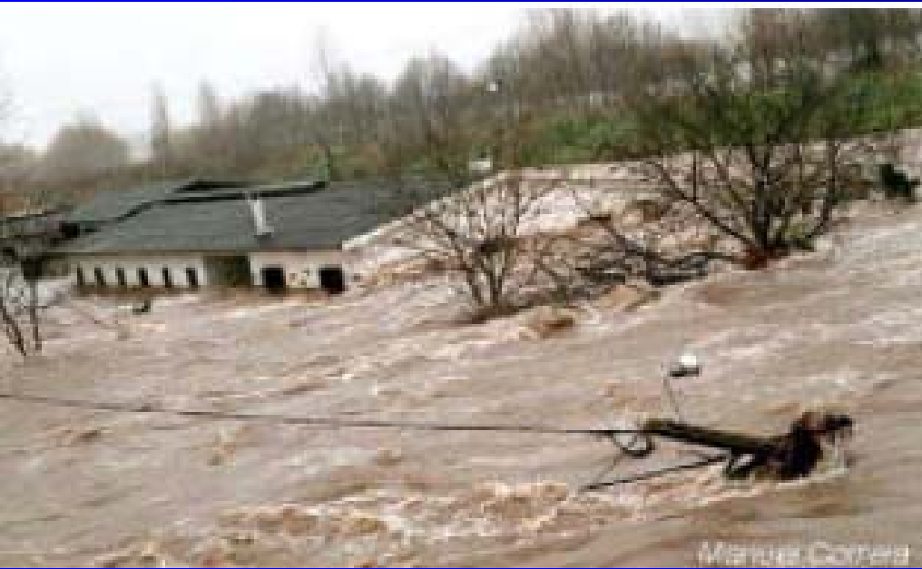
Damage to lifeline systems Portugal, 2001
