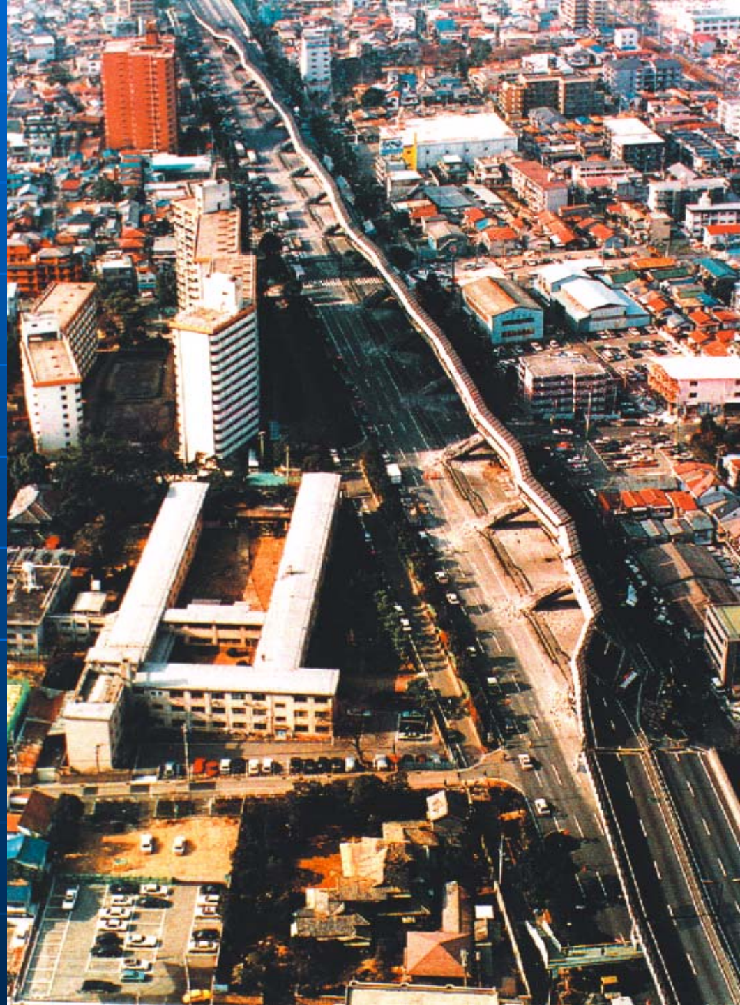
Elevated highway damaged during the Hanshin – Kobe 1985 EQ. (Photo Nakanihon Air Service Co. Ltd.)
