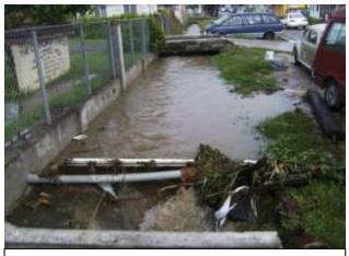
Fig: 42 Littering/illegal dumping blocking drains Source: NODS
