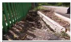
Fig: 35 Potential road undermine and collapse: Source NODS
