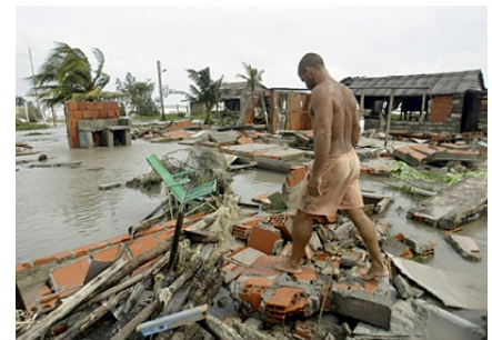
Severe damage after a hurricane. IFRC.
