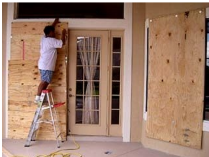
Preparations for hurricane winds.
