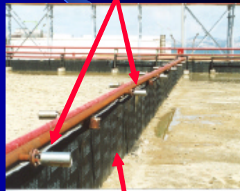
Containment dike liner installed after the earthquake.
